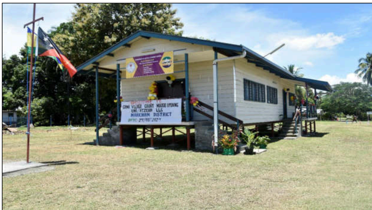
Figure 29. Gama/Zu Village Court House in Morobe Province, is one of the selected Village Court Areas to see the first ever VC House constructed and built at Mutzing Station. It was completed and commissioned on March 29th 2024.
